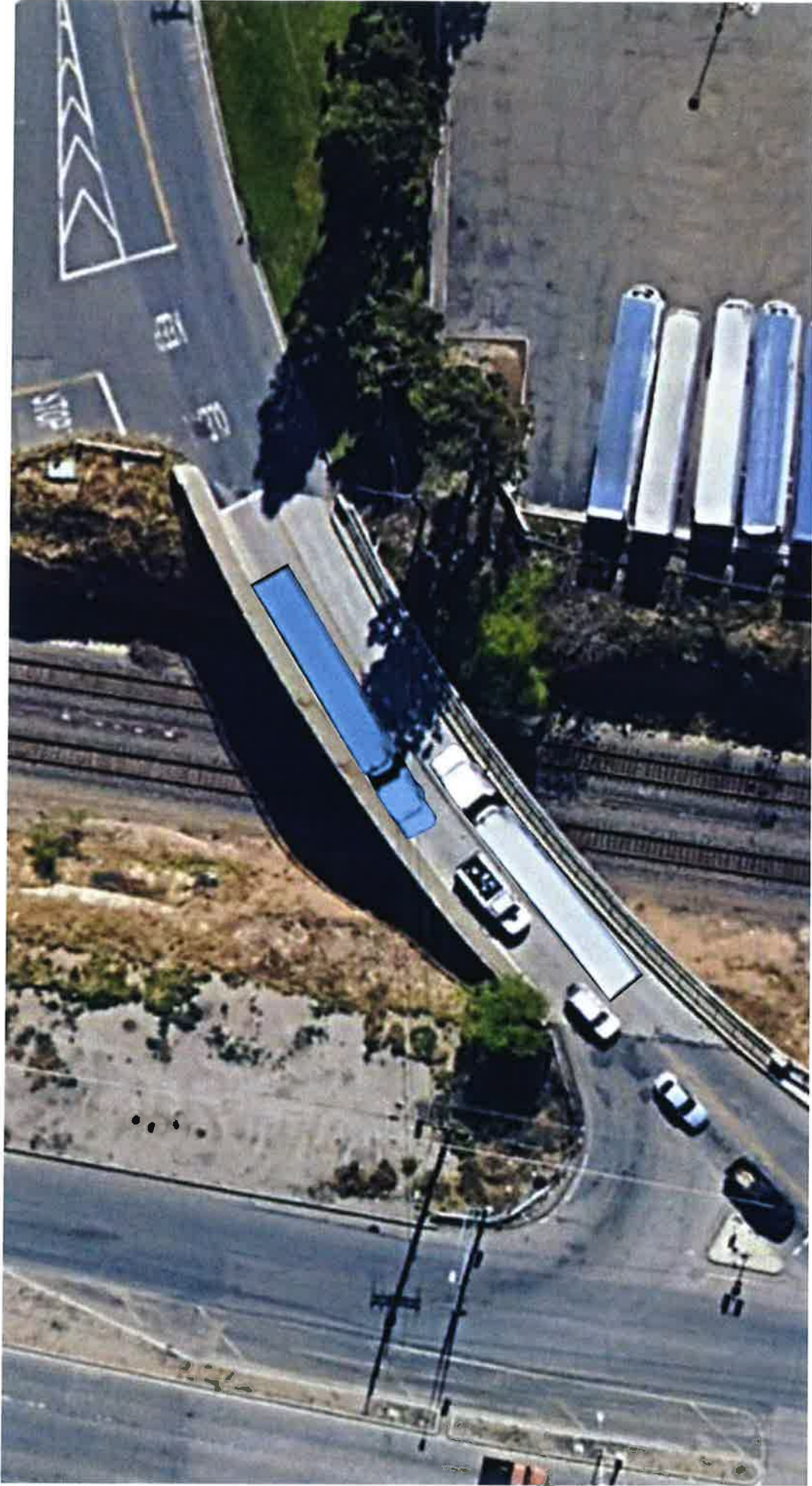
Exhibit 1 Existing Barton Road Across the Bridge Over the BNSF tracks
